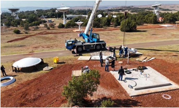
Figure 20: AIRCAS expansion construction
