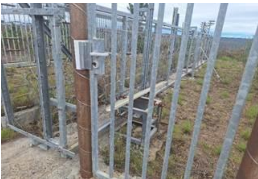
Figure 7: Gate motor at Houwteq
