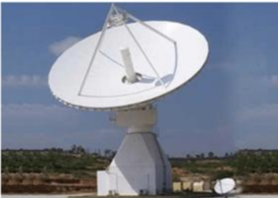
Plate 3-2: LGS18, Ka Antennae, 18m wide dish, 30m height.
