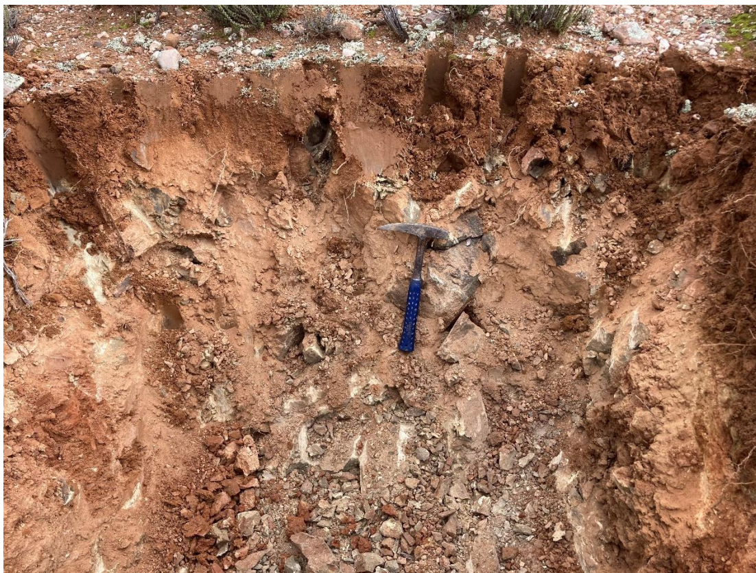
Figure 48 SMTP24 test pit excavations
