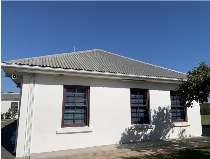
Figure 1. Roof space for installation of PV panels.
