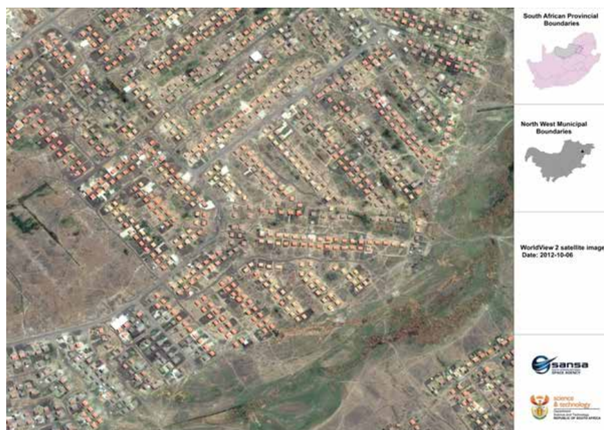
Figure 6: Seraleng Low-cost housing development.
